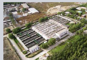
Waste water treatment Beixiaohe
